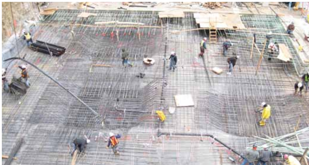
Figure 1. Mat foundation for a building under construction.
