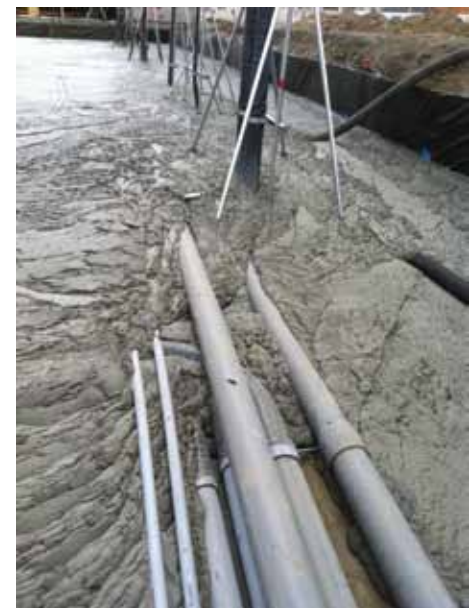
Cellular concrete flows into every nook and cranny with no vibration or placement effort.
