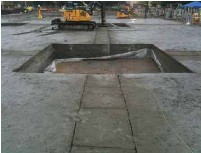
Lightweight foundation fills that are excavatable yet placed cost effectively and extremely fast.
