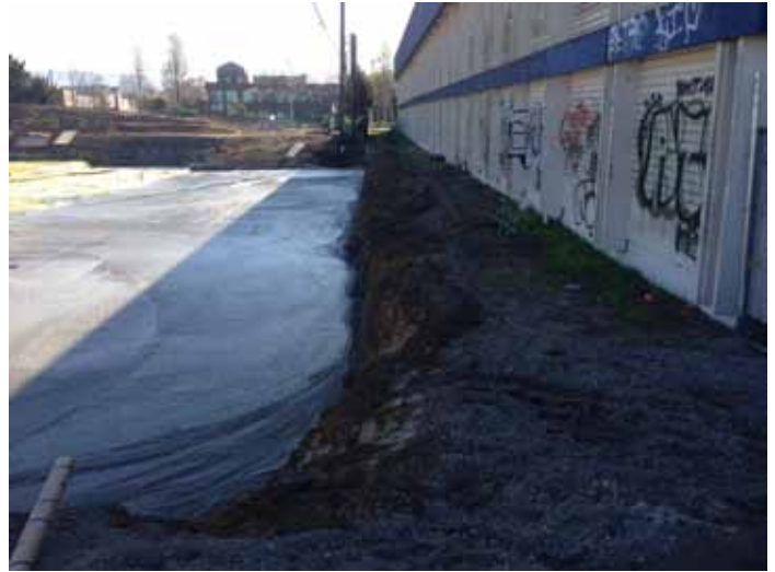
Load balancing fills adjacent to existing structures do not cause adverse movement.
