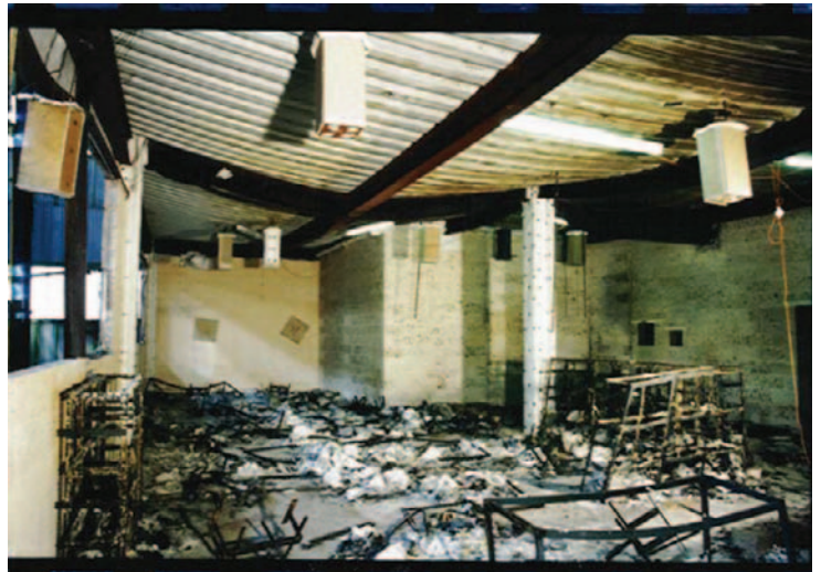
Floor, Full-Scale Fire Test (Cardington, UK)
