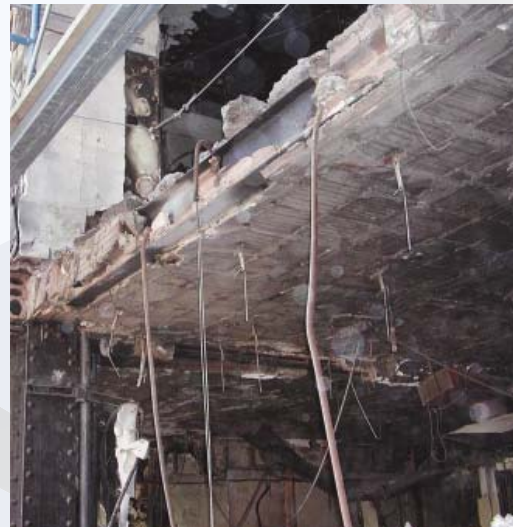
Figure 6 – Flat arch tile floors in 90 West Street
