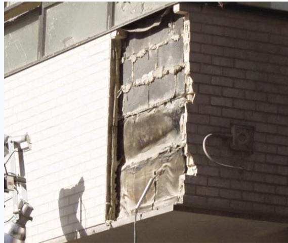
Figure 5 – Southeast corner of 30 West Broadway
