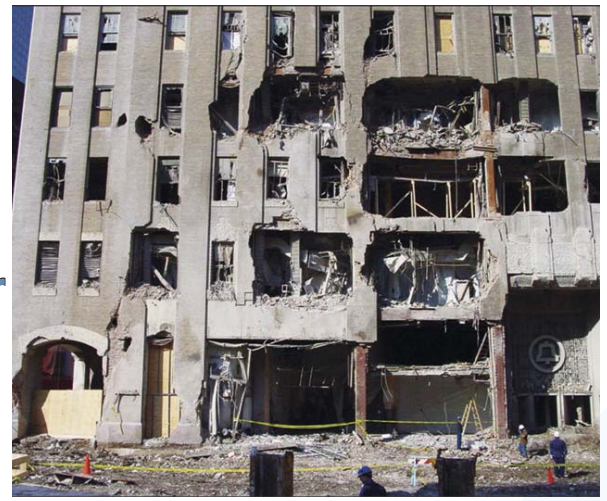
Figure 2 – East elevation of 140 West Street
