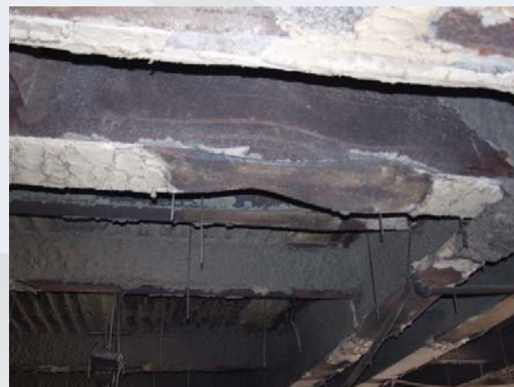
Figure 7 – Floor framing in WTC5
