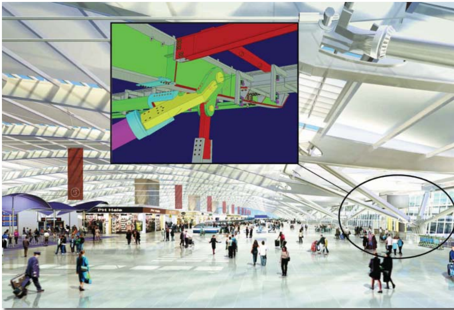
“Over the past three years the British Airport Authority team has been using Tekla products on the Heathrow Terminal 5 (T5) project in London. T5 is the UK’s largest construction project and is due to be completed in 2008. (‘Top-Down’ technology has) allowed 3D Structural Steelwork model collaboration between T5 design team members, while at the same time utilizing and developing the steelwork contractor’s production model” - Nigel Bradley BAA 3D Cad Coordinator. Heathrow Terminal 5
