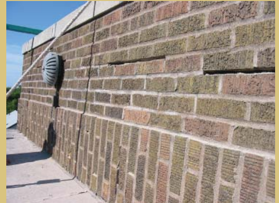
Figure 2: Close visual inspection of the same parapet shown in Figure No. 1
