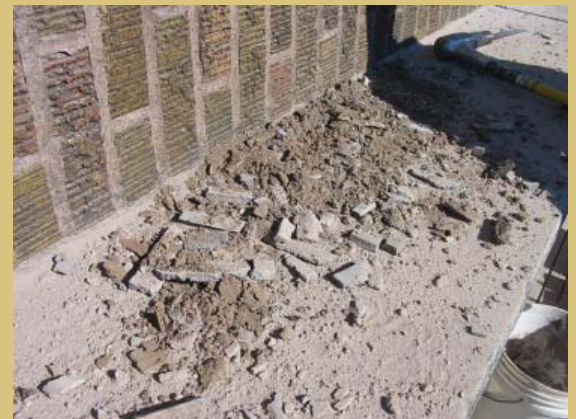
Figure 3: Damp inner wythe mortar material from test opening at same location
