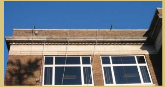
Figure 1: View from grade of the three-story building parapet
