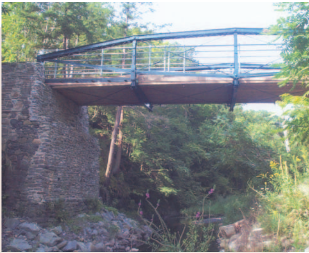
Bridge at Malta, August 2003
