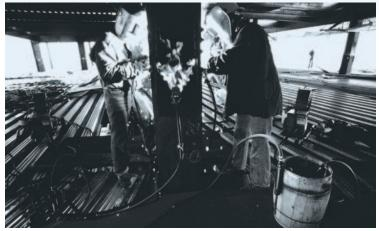
Maintaining specified preheat and interpass temperatures is essential to ensuring the proper performance of welded connections.
