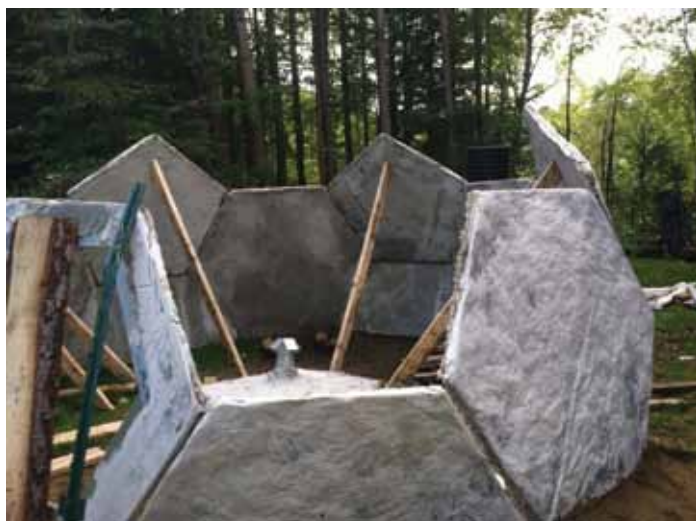
Figure 5. Temporary supported 2 nd level. Courtesy of Megan Strand-Jordan.
