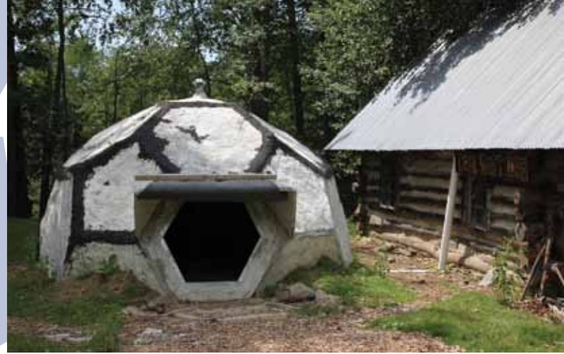
Figure 1. Completed structure. Courtesy of Meghan Holland.
