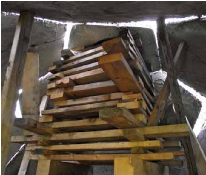
Figure 7. Inside view of interior cribbing/scaffolding. Courtesy of Megan Strand-Jordan.
