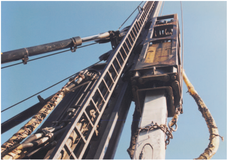
Driving a pre-stressed concrete pile with a hydraulic hammer.
