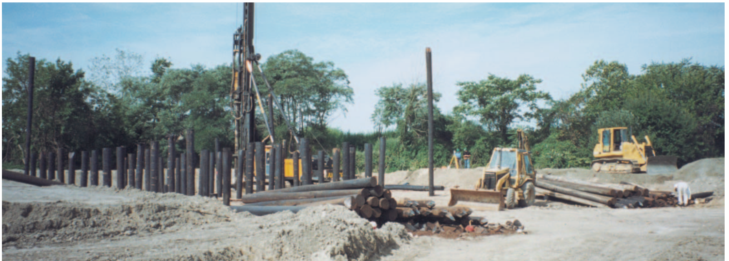
Driving timber piles with a hydraulic hammer.
