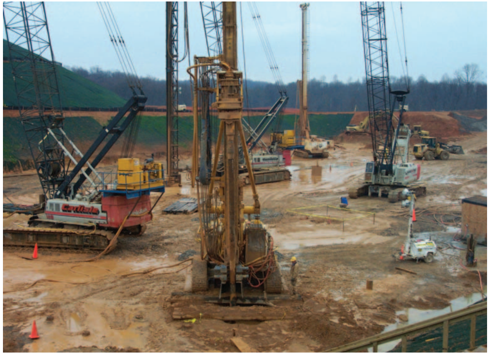
Baur BG-22 Drill Rig and Fixed Lead Crane Attachment Drills
