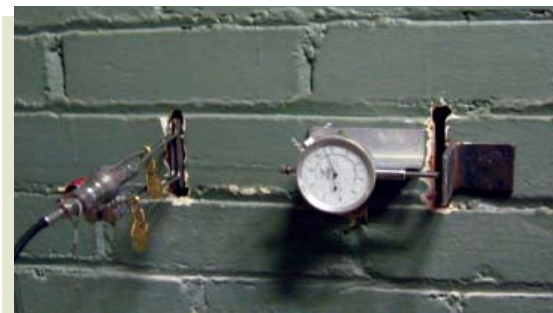
Figure 10: An in-place shear test, conducted here using a small flatjack inserted into a cleared head joint. The force required to displace the test brick (thus shearing the mortar joints above and below) is used to calculate masonry shear strength.
