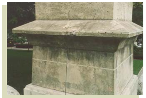
Figure 4: View of stone imaged using tomographic methods; the horizontal cross section shown below is marked with masking tape on the stone.
