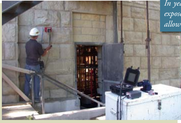
Figure 1: Radar scanning of an historic stone wall.
