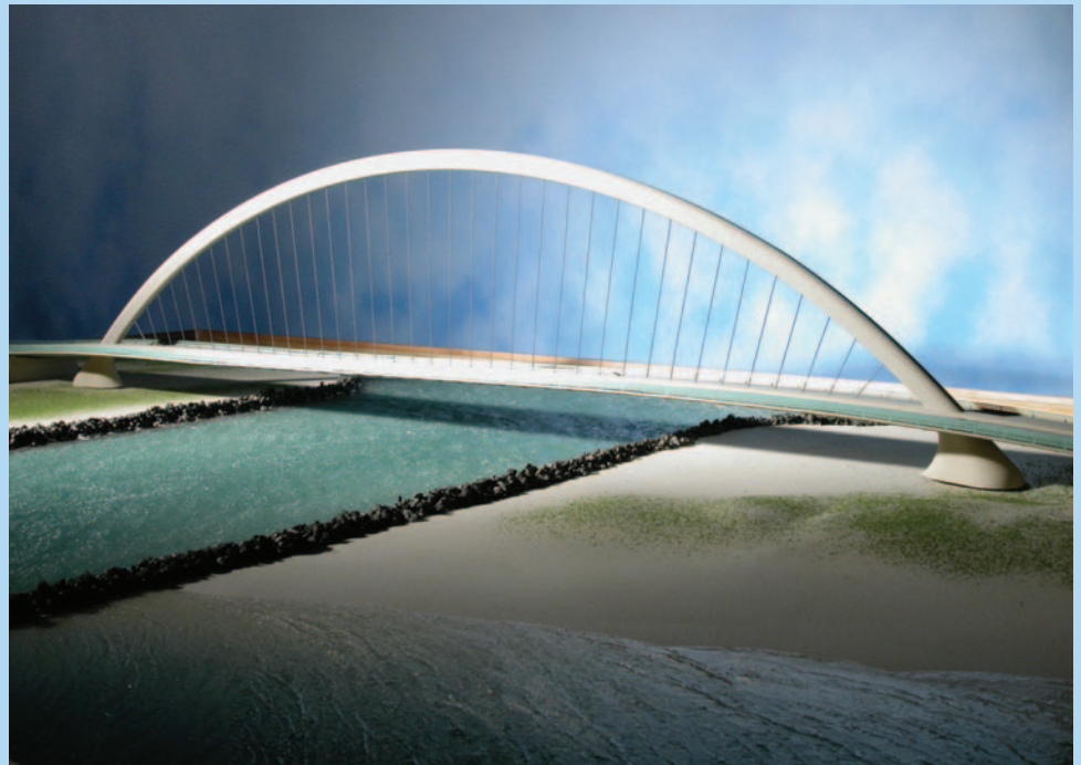
The grand, sweeping arch rises from the ocean shoreline dunes. The arch, with its single plane of radial stays, supports a 1000-foot span across the waterway, avoiding the need for piers in the inlet.
