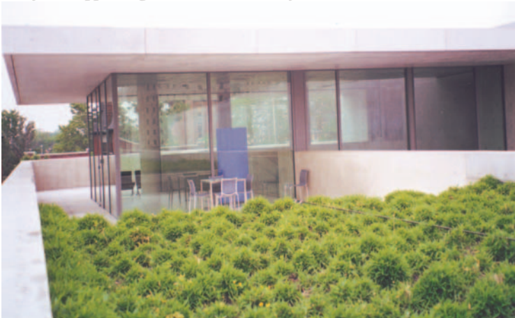
Pictured above: The two-way cantilevered roof was required to be perfectly level (showing completion).
