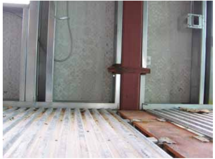
Figure 4. The 10-story Convent Hill senior housing complex features a new level of sustainable and green technology.
