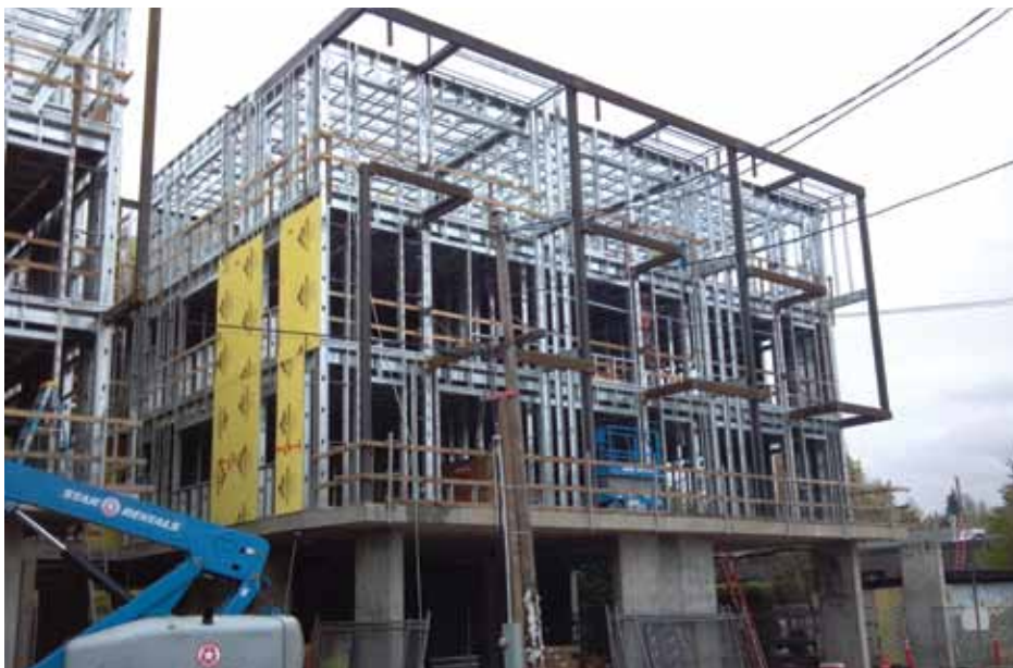
Figure 4. Cold-formed steel framed building. Courtesy of Equilibrium Engineers, LLC.
