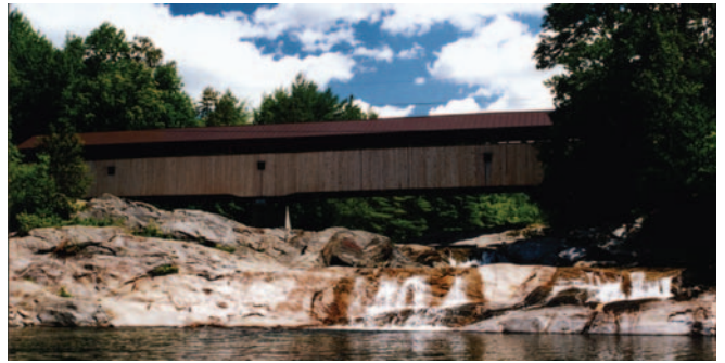
Swiftwater Covered Bridge, Bath, NH
