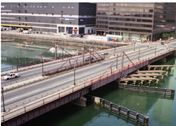
Summer Street slider system bridge
