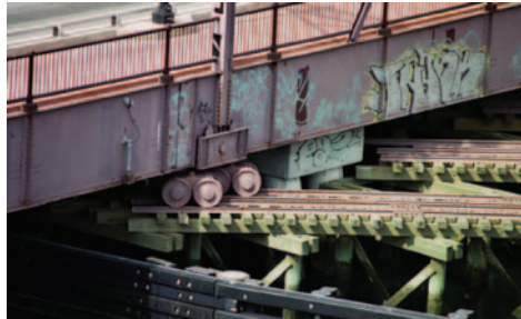
Summer Street Bridge slider system detail
