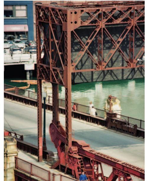
Congress Street Bridge detail of bascule system
