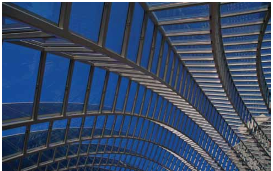
Figure 7. Expansion bolts secure the stunning HSS-framed roof at The Kimmel Center for the Performing Arts in Philadelphia.
