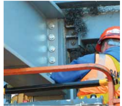
Figure 5. Expansion bolts are quick and easy to install.
