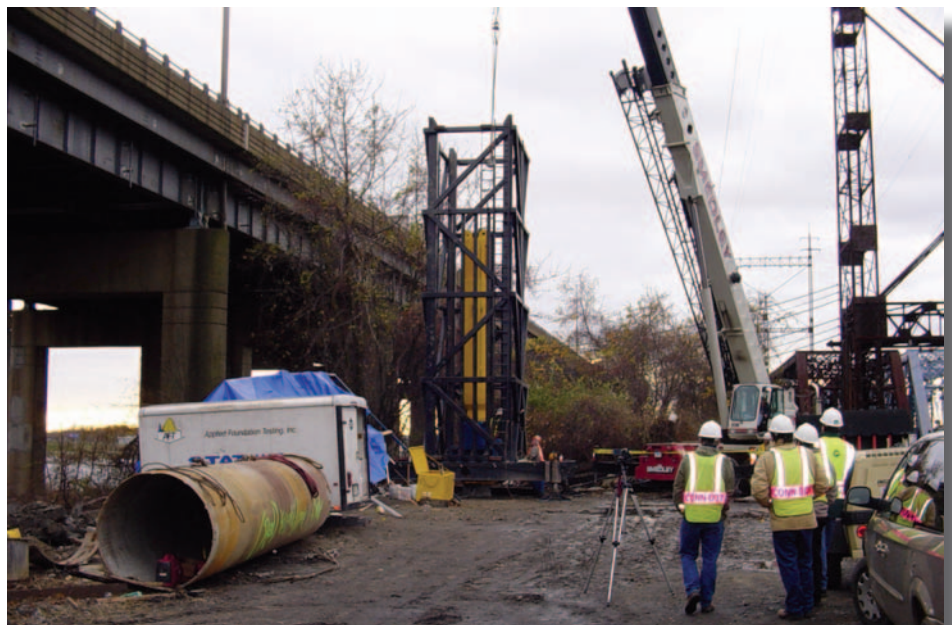
Figure 4: 2000 Ton Statnamic Device with Mechanical Catching System, Stratford, CT
