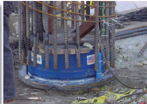
Figure 6: O-cell attached to drilled shaft enforcing cage, Stratford, CT
