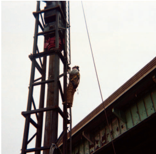
Figure 3: Attaching PDA Sensors to a Driven Pile for Dynamic Testing
