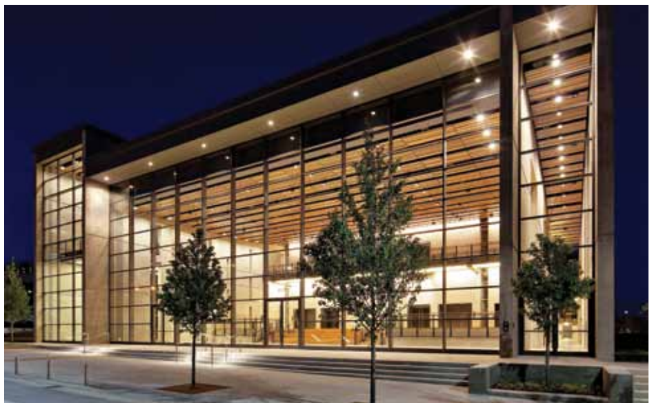
Steel's greater load carrying capacity allows building teams to increase glass sizes in steel frames.
