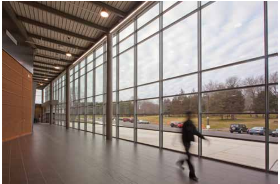
Steel veneers allow for attachment to virtually any structural component that can support the curtain wall system's imposed loads.
