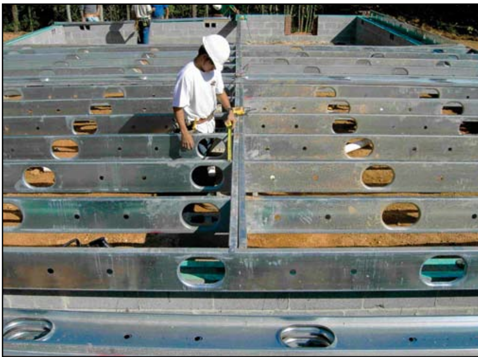
Several manufacturers have floor joist systems with large, stiffened (lipped) holes, which facilitate the installation of MEP services. Other components of these systems include rim tracks with tabs for connections and stiffening, and engineered tracks that can span moderate wall openings without headers.
