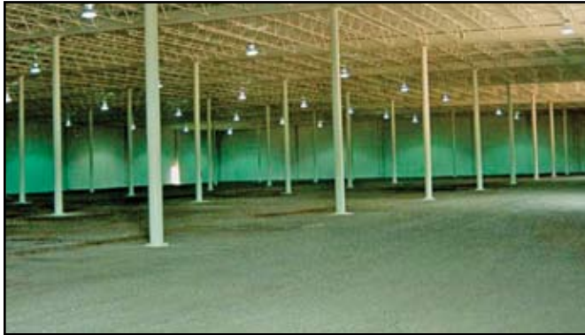
Figure 1: A perfect world – an industrial shell building ready for slab installation
