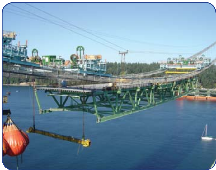
Lifting Gantries and Erection of Structure Segments at Midspan
