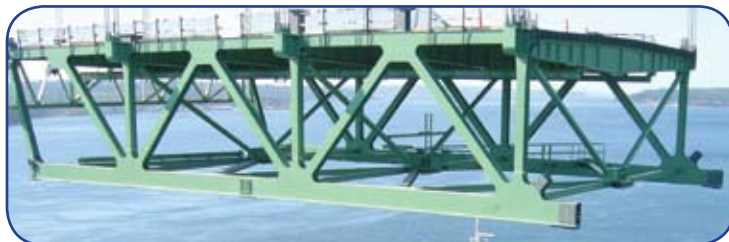
Structure Segment lifted from Transport Vessel
