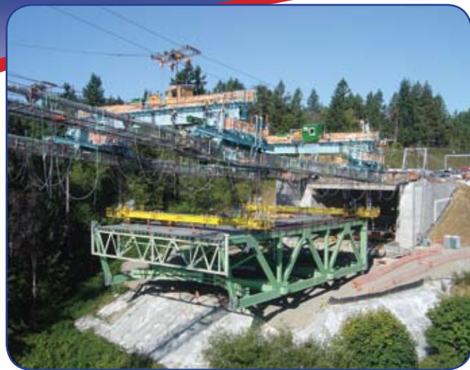
Trapezing Segment 1 to Gig Harbor Anchorage
