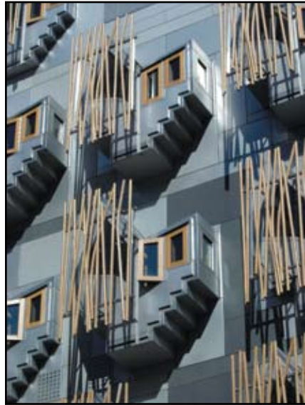
Figure 1: Blast-resistant Windows in the Scottish Parliament Building. ©Arup
