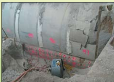
Figure 4: Demolition of damaged knee wall
