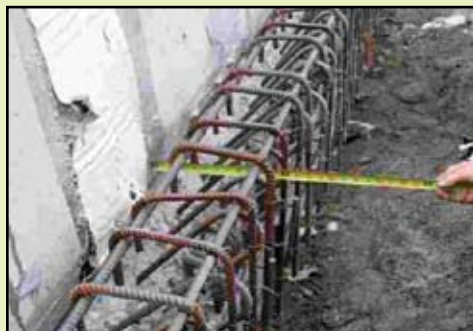
Figure 5: New knee wall reinforcing steel
