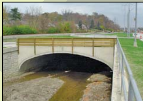
The Completed culvert
