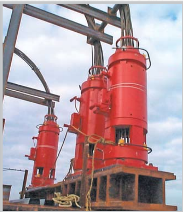
Figure 5: Strand Jack Heavy Lift Technology.
