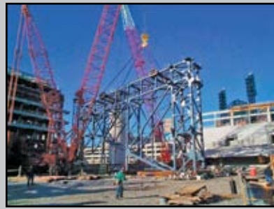
Tip up of truss assemblies
