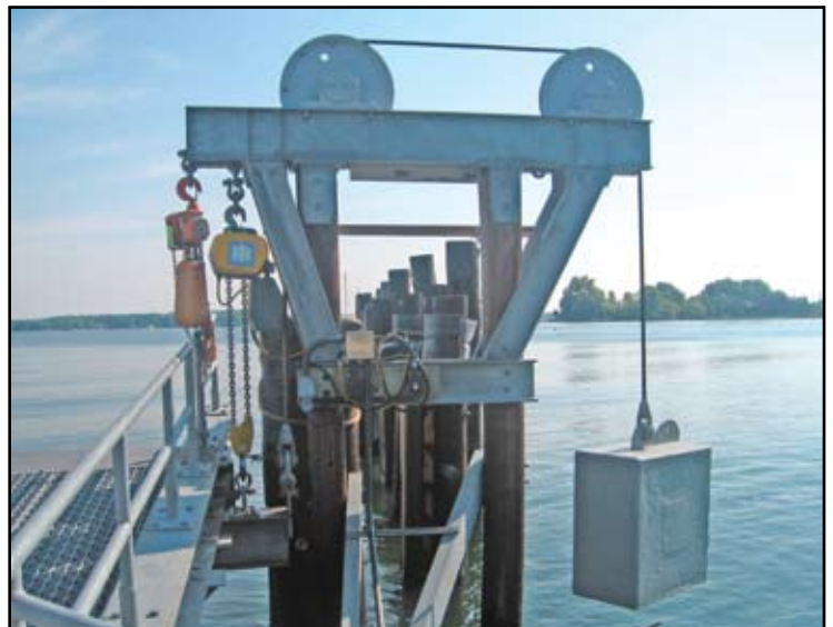
Figure 4: New components on south hoist tower
