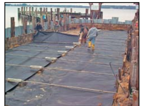
Figure 6: Back-to-back tiebacks for steel sheet piling on approach roadway
