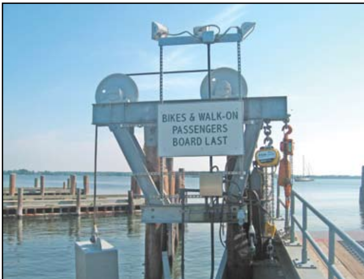
Figure 3: New components on north hoist tower
