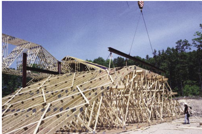
Large trusses set in blocks, assembled and braced on the ground.
