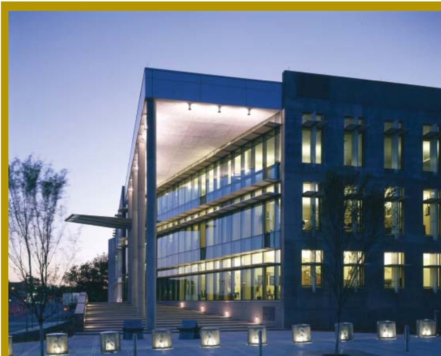
Figure 5: Balanced blast design can yield a light, but blast-worthy curtainwalls
