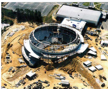
Crown Center Construction
