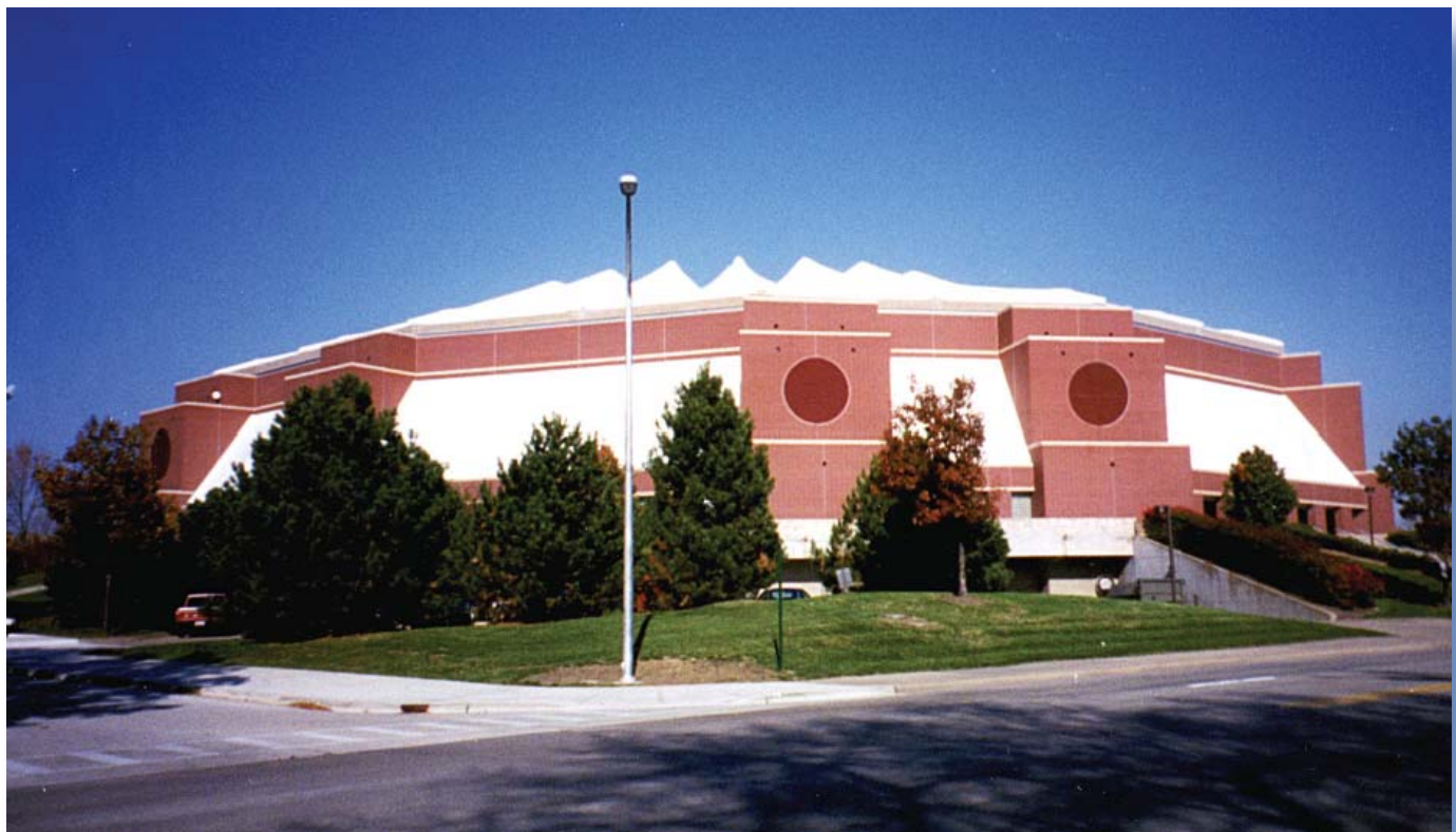
Redbird Arena, ISU, Normal, IL: 1988-First Cabledome in USA clad with pleated fabric membrane
