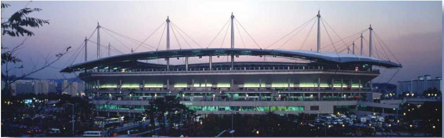
Seoul 2002 World Cup Stadium: Canopy cable suspended from 16 masts
