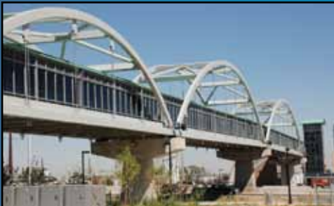
Hwy 36 Bridge Denver, CO.
