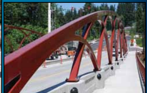
May Creek Bridge Redmond, WA.
