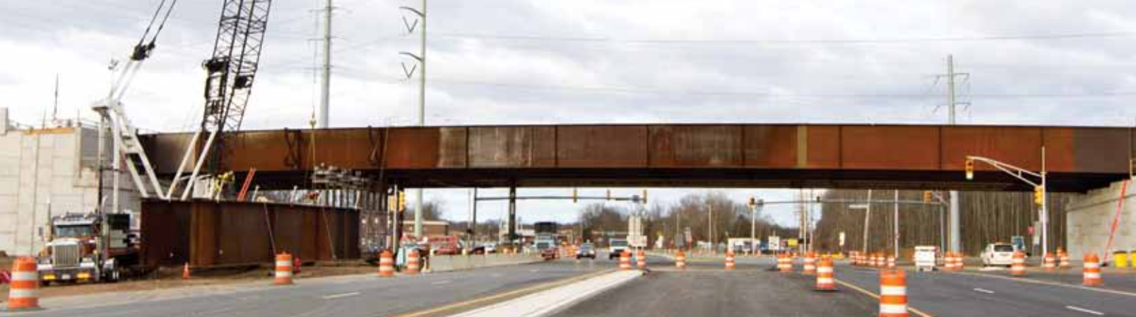
Figure 5. Erected Girder Lines 1-4 with jack posts in place.
