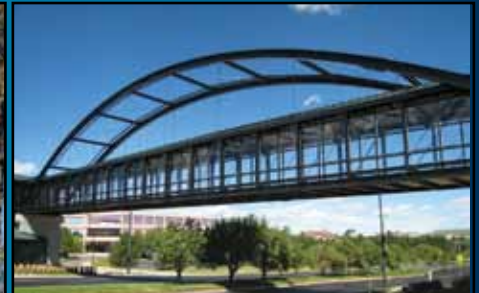
Dry Creek Bridge Denver, CO.
