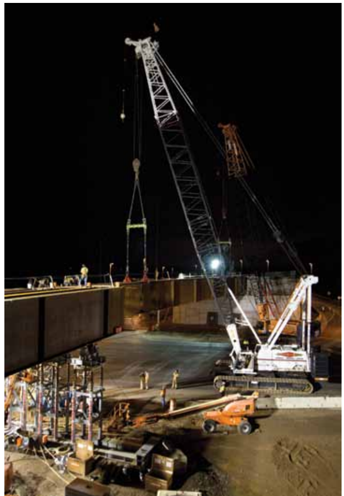
Figure 2. Erecting Girder Pair A/B.
