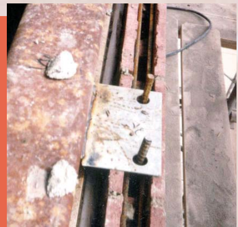
Figure 6: Structural Brick Veneer Connector
