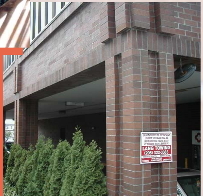
Figure 8: Brick Wall for Gunite Backup
