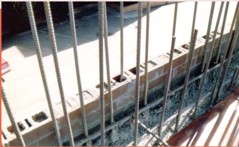
Figure 9: Brick Panels as Concrete Forms
