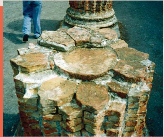
Figure 2: Fluted Roman Brick Column
