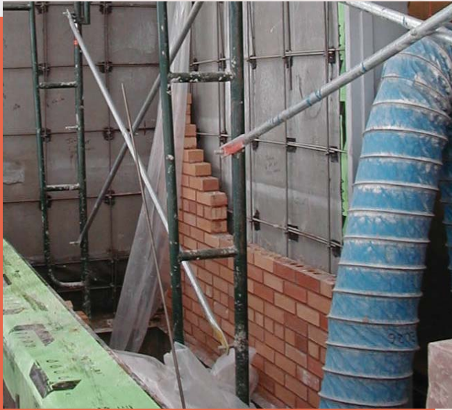
Figure 7: Reinforced Veneer on Steel Studs Before Grouting
