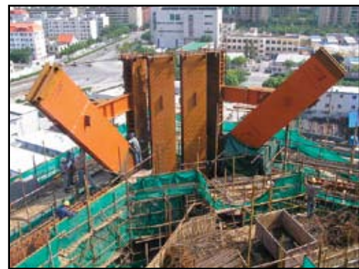
Figure 4: Mega Column/Mega Diagonal.
