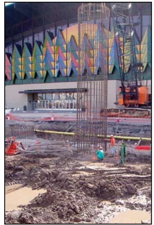
40-foot deep drilled piers at Hydraulic Canal
