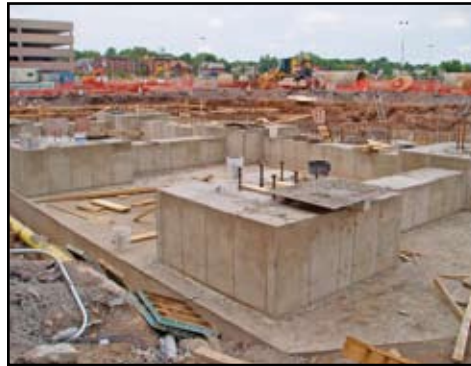
Concrete grade beams and pier caps above structural mat
