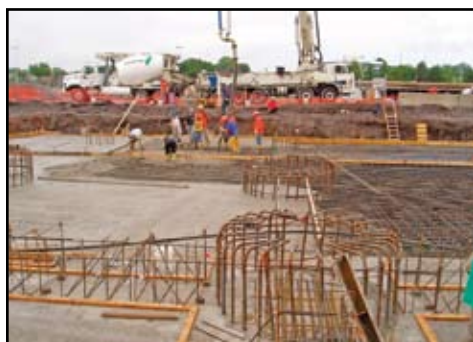
Placing concrete in the mat
