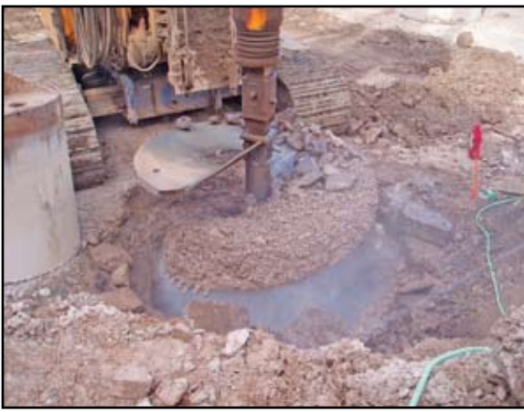
9-foot diameter drilled piers
