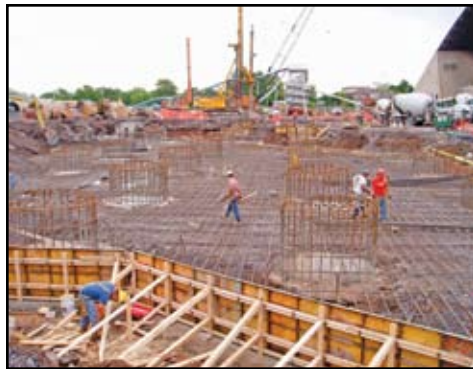
Structural mat and drilled piers over the Hydraulic Canal
