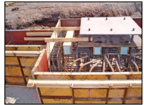
Anchor bolts and shear keys set into pier cap
