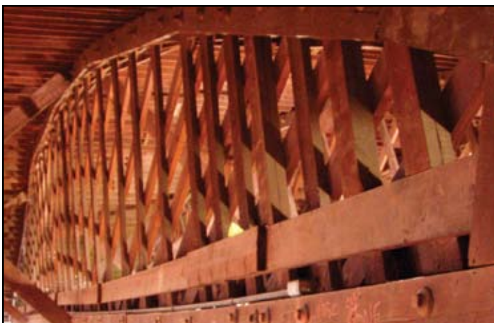
Figure 2: Curved-chord wooden lattice trusses support the roof of MIT's W33 Cage Building.
