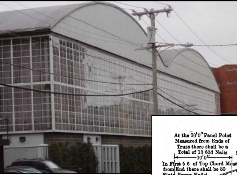
Figure 1: Double-barrel vault roof profile of MIT's W33 Cage Building.
