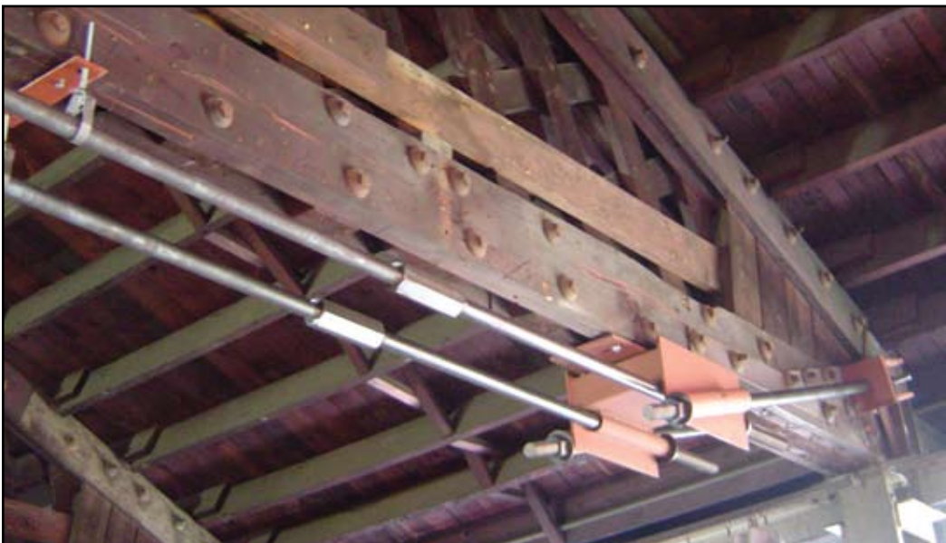
Figure 3: Lower bracket transfers tension from diagonal tie-rods into horizontal tie-rods.
