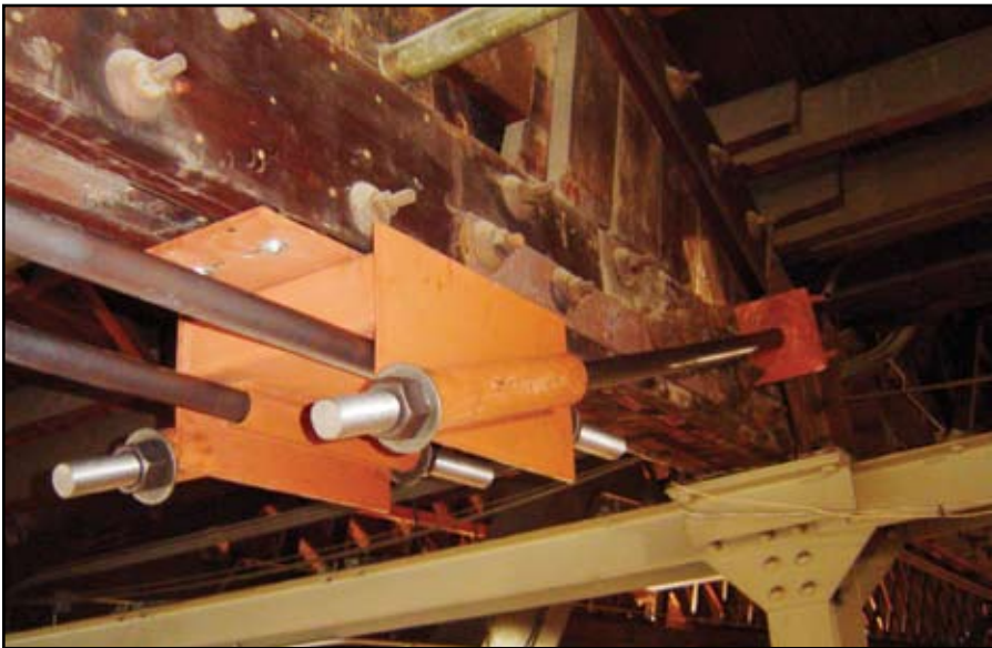
Figure 3: Lower bracket transfers tension from diagonal tie-rods into horizontal tie-rods.
