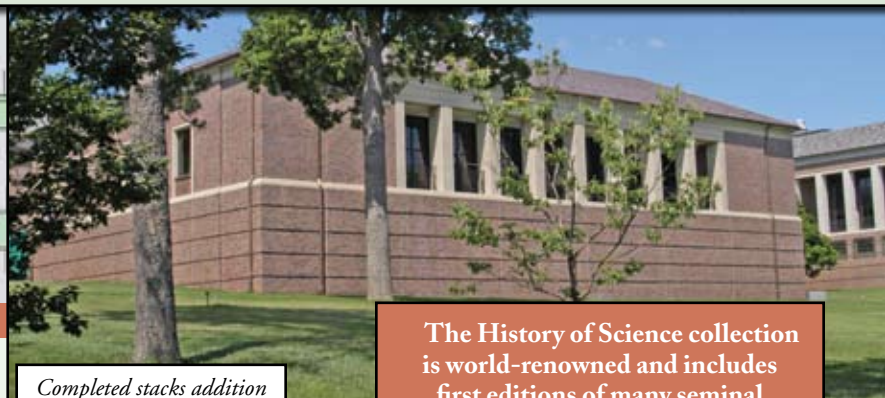
Completed stacks addition
