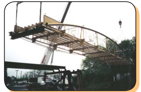
"Flight of the Phoenix" — rehabilitated bridge being lowered into place
