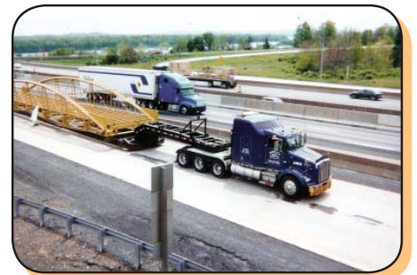
Rehabilitated bridge enroute to Summerdale Campus
