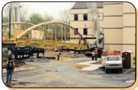
Bridge being lowered into place
