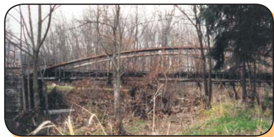
Side view of arch on its abutments before lifting
