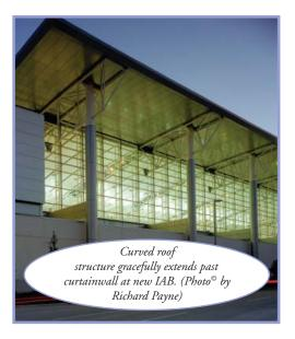
horizontal and located directly behind the curtain wall mullions. We designed 8.625-inch diameter pipes to support the vertical loads.
