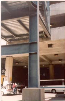
Figure 2: Steel Column Protected with Epoxy Based Intumescent (Photo Courtesy of PPG Industries, Inc.)
