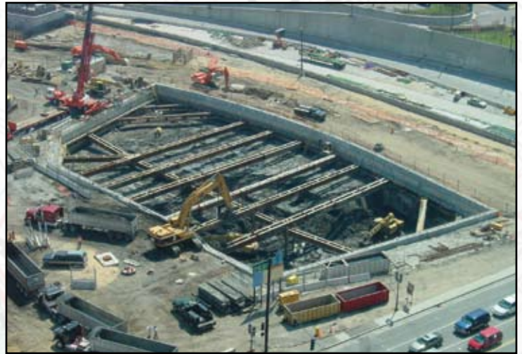
Manulife project during staged excavation and mat foundation construction
