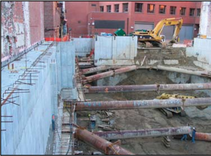
Diaphragm wall bracing installation at the Piano Row site
