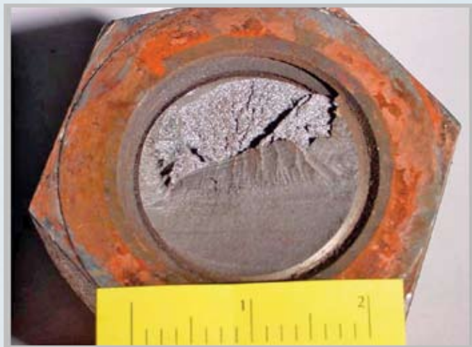
Figure 4a: Fatigue fracture of a structural steel bolt. Note fracture is characterized by a smooth dull appearance and beach marks.
