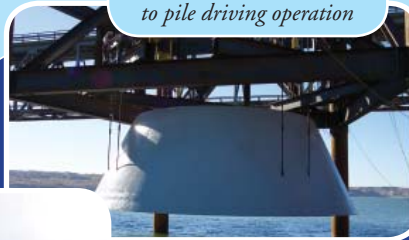
36-inch steel encased concrete pile support pier footing, cofferdam and pier
