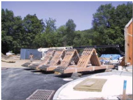
Typical truss half sub-assemblies. Note symmetric geometry. ©Bridgeport Design Group
