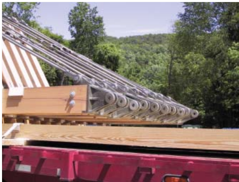
Typical truss top chord end fitting. ©Bridgeport Design Group
