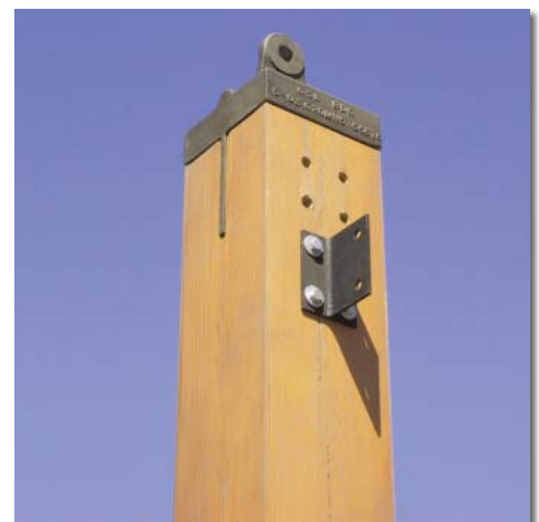
Typical column head fitting. ©Bridgeport Design Group
