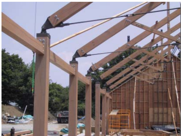
Assembled roof trusses in place, showing supports. ©Bridgeport Design Group
