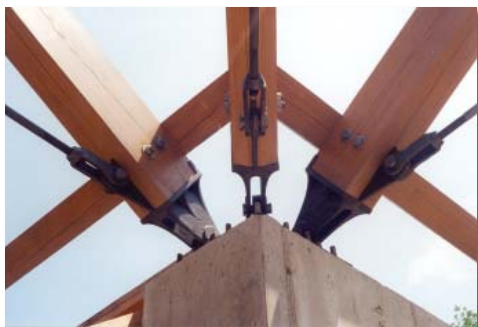
Roof truss support fittings at 3 dimensional truss support.
