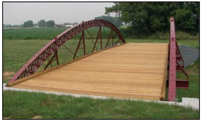
Figure 6: Relocated bridge prior to trail construction and railing installation.
