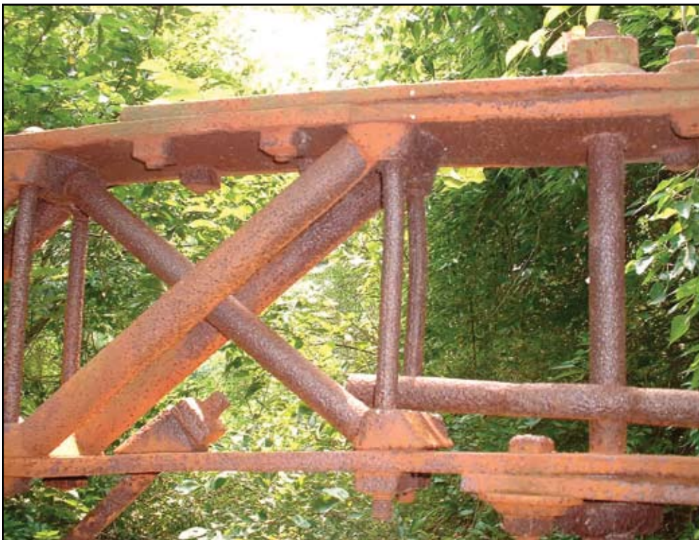
Figure 2: Arch detail at mid-span splice prior to rehabilitation.
