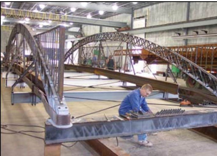
Figure 4: Bridge under rehabilitation at Ohio Bridge Corp.
