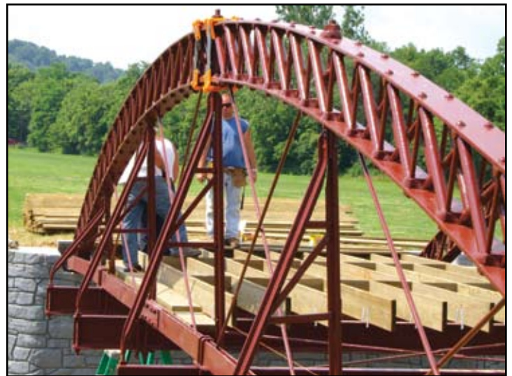
Figure 5: Relocated bridge receiving deck.
