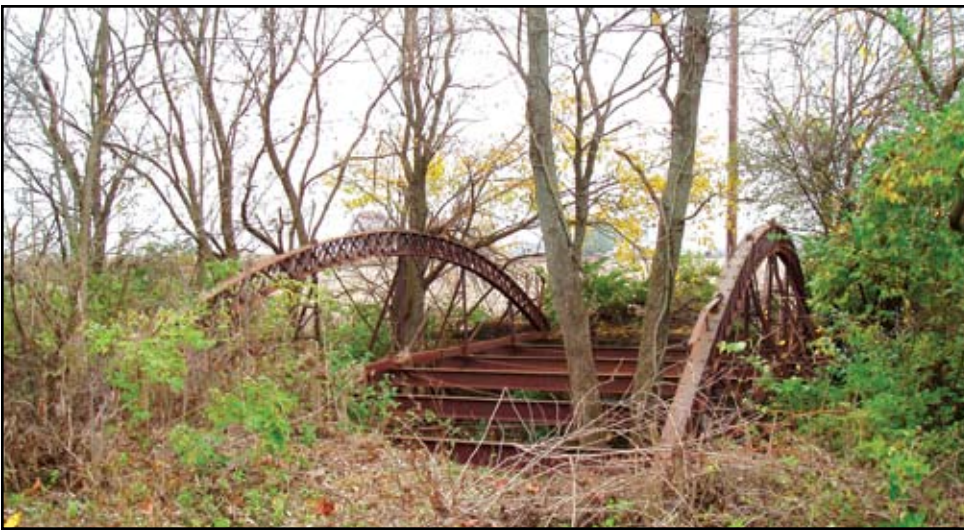
Figure 3: Structure as discovered adjacent to Oxford Road.
