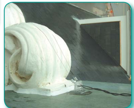
Electric wires — birds remember and avoid locations of electric shock. Photo by Michael Teller, CBI Consulting, Inc.
