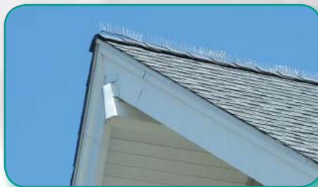
Spikes eliminate places to land, loaf or walk. Photo by Michael Teller, CBI Consulting, Inc.
