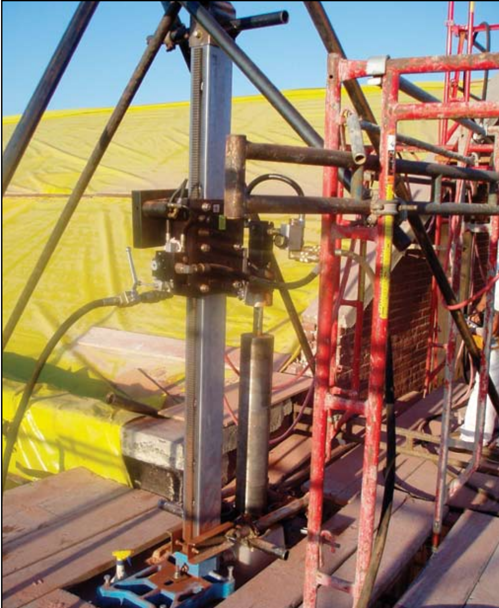
Coring Operation in Brick Wall. Courtesy of Cintec North America.
