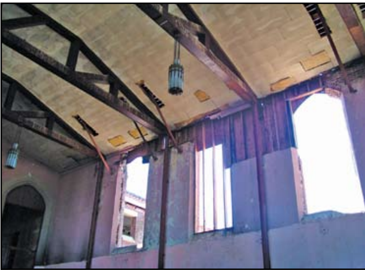
Interior Showing Roof Truss and Prior Retrofit Posts and Wall Anchors.
