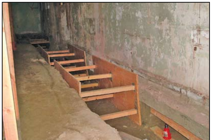
Formwork for New Foundation.
