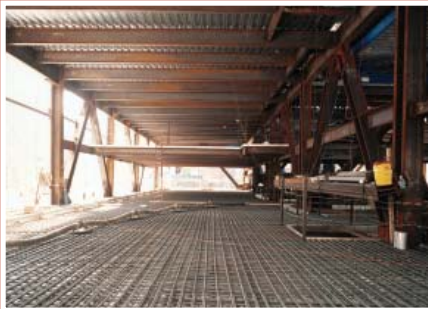
Reinforcing in slab to connect belt trusses to core bracing
