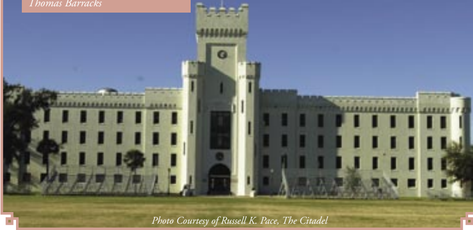
Front view of the completed Padgett-Thomas Barracks
