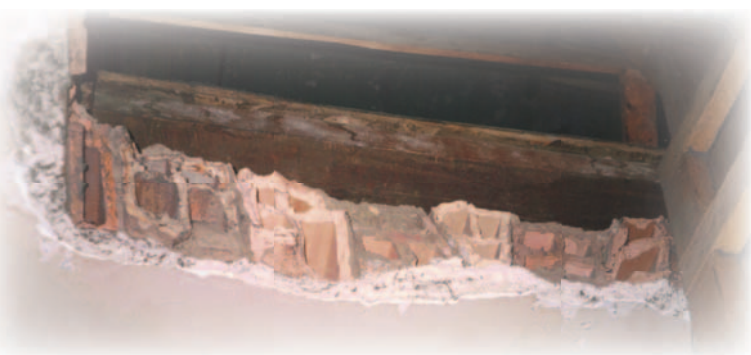
Photograph of hole cut through tile arch floor.
