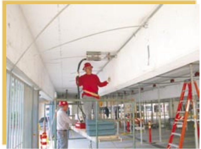
Stressing external tendons in an existing structure
