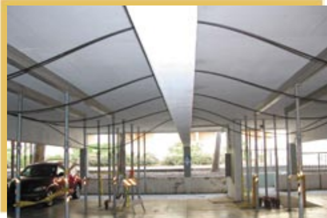
Unstressed external slab tendons
