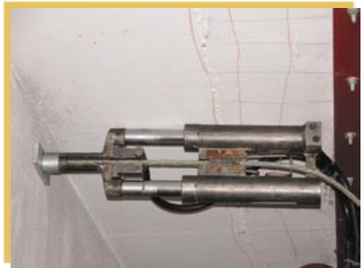
Close-up of the jack stressing the tendons
