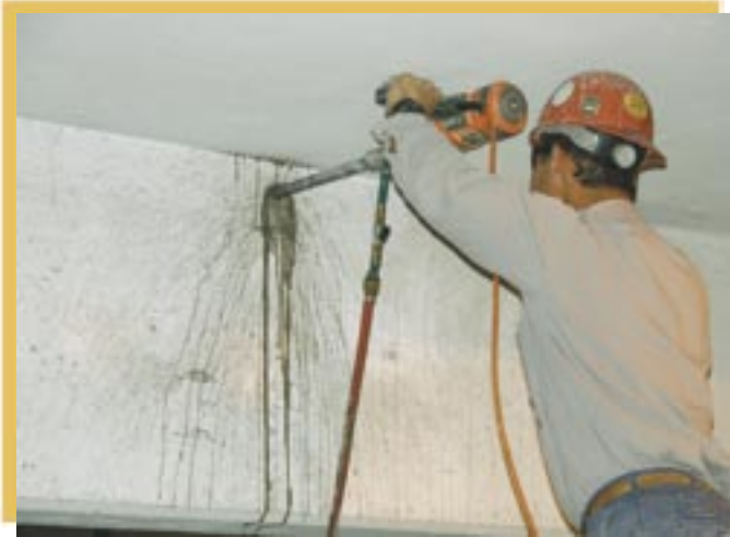
Coring through an existing beam
