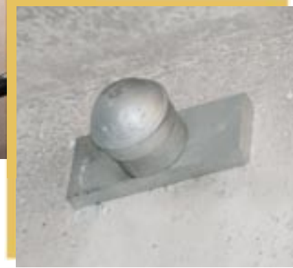
Galvanized anchor plate, barrel anchor and cap
